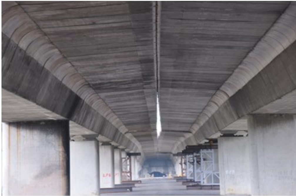
Figure 6. Maximum lateral displacement of 55 cm in the bridge deck and box girders of the left bridge equipped with seismic isolation pads, relative to the corresponding elements of the right bridge.
