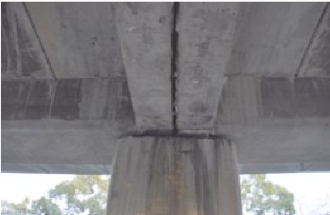
(b) Transverse view of the bridge.
