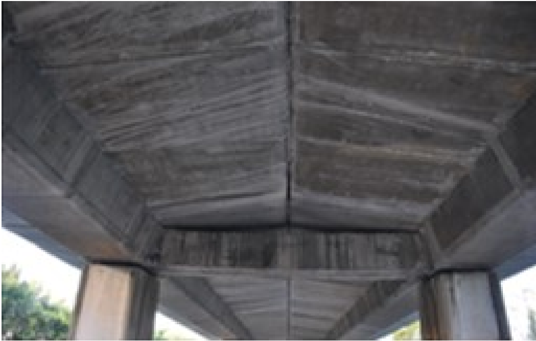
(a) Longitudinal view of the bridge.
