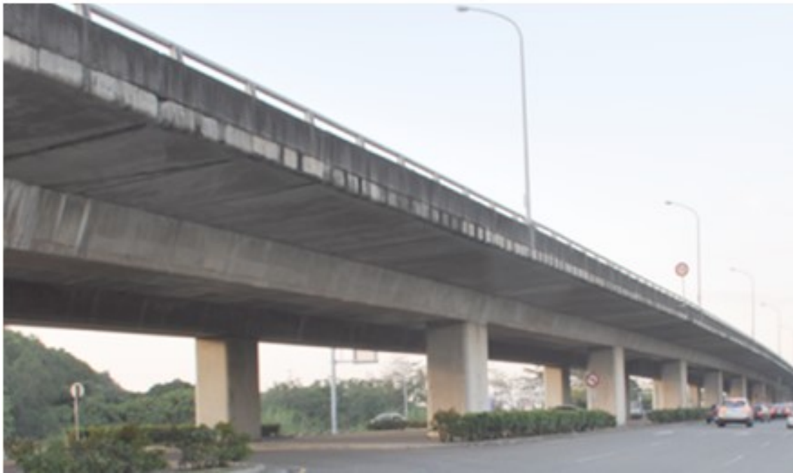
Figure 1. Land bridge on Highway Tai-86 in Tainan, Taiwan.
