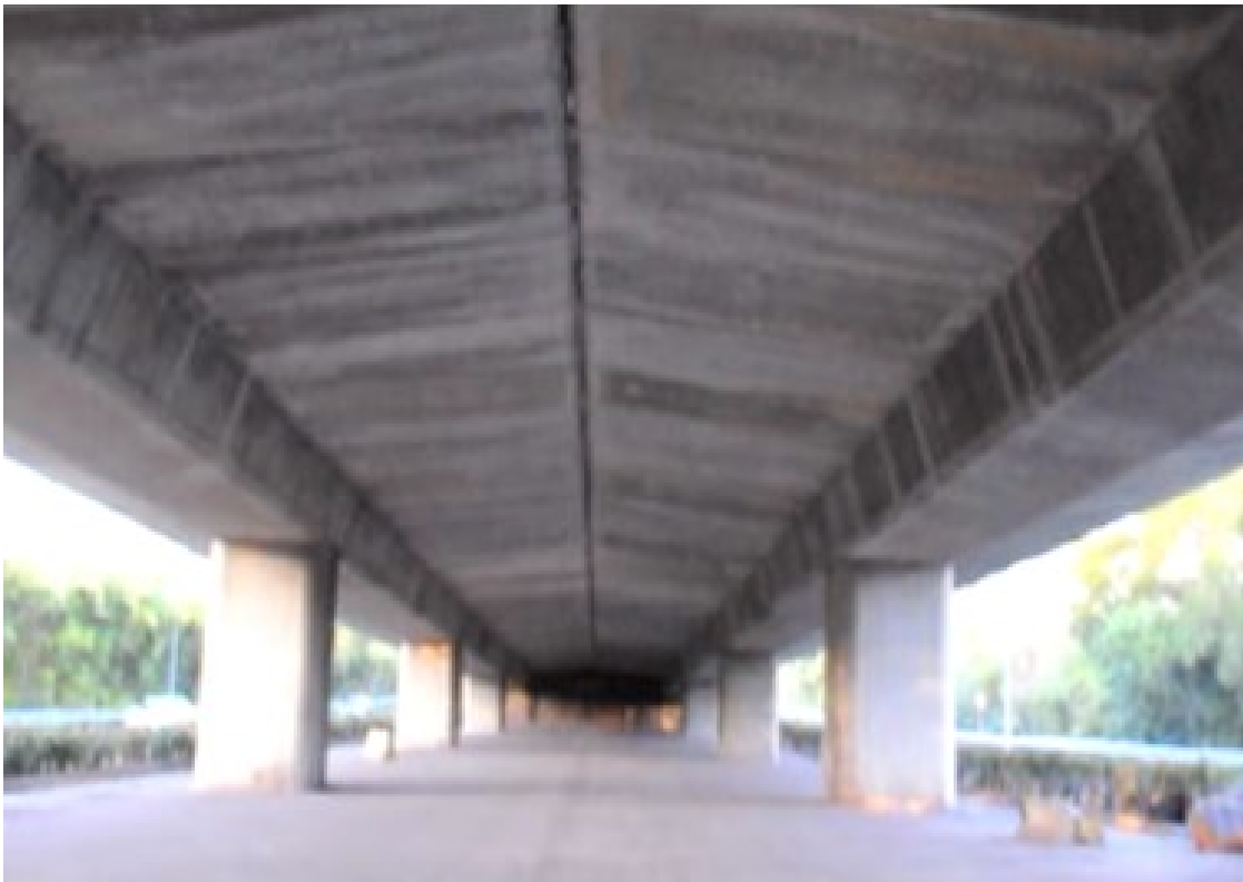
Figure 4. Absence of shear banding on the ground adjacent to the piers of the land bridge without isolation pads.
